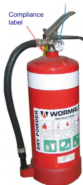
Figure 81.1 Fire extinguisher compliance details Wet Paper
